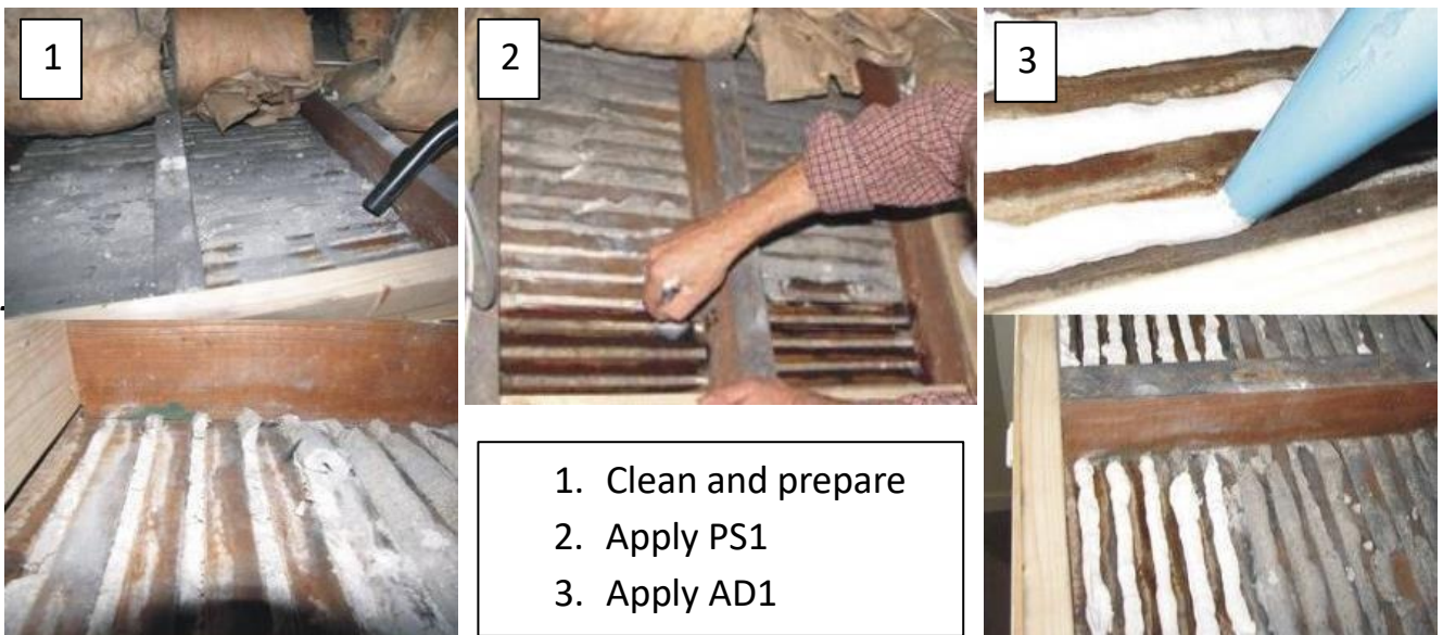
Application on damaged or loose panels
